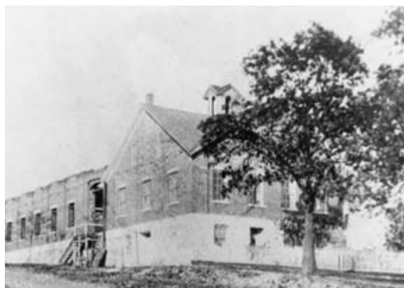
A house built on the foundation of the original Nauvoo House, with original north wing
